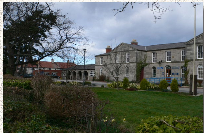
H.M Stanley Hospital, St Asaph, Denbigshire
